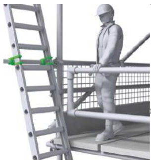
✓ Figure 9 Correct – access ladders should be tied and extend at least 1 m above the landing point to provide a secure handhold
